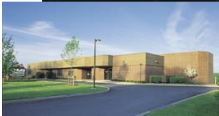
▲ CMI's Main Campus at the Utica Business Park
